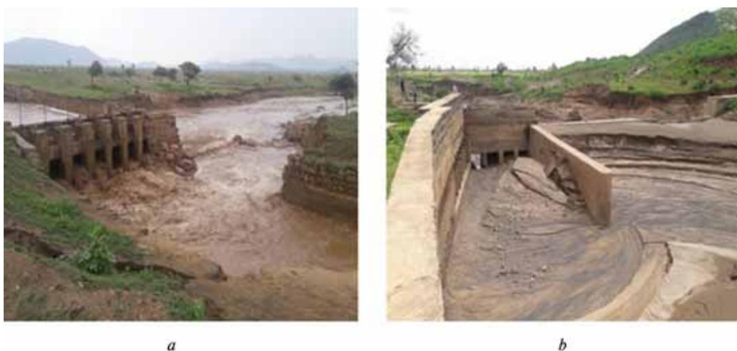
Fig. 2. Complete and partial failure of the irrigation diversion structures in Hashenkit (a) and Golij-Ingulit (b)
