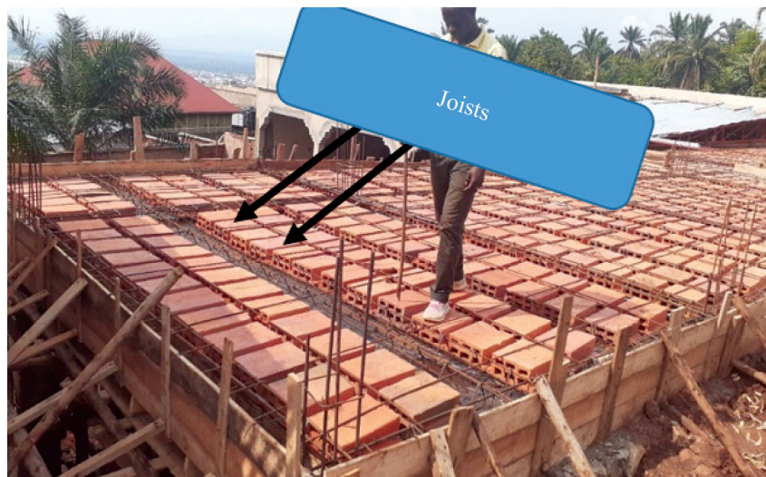
Fig. 1. Photo illustrating a slab with joists in a reinforced concrete building under construction in Burundi
